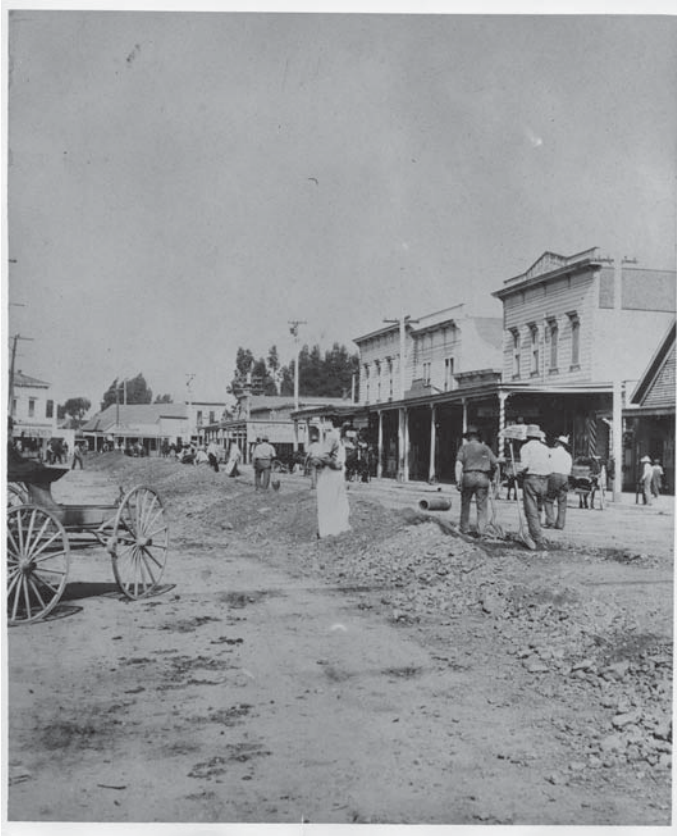
Installing sewer pipe on First Street circa 1904
