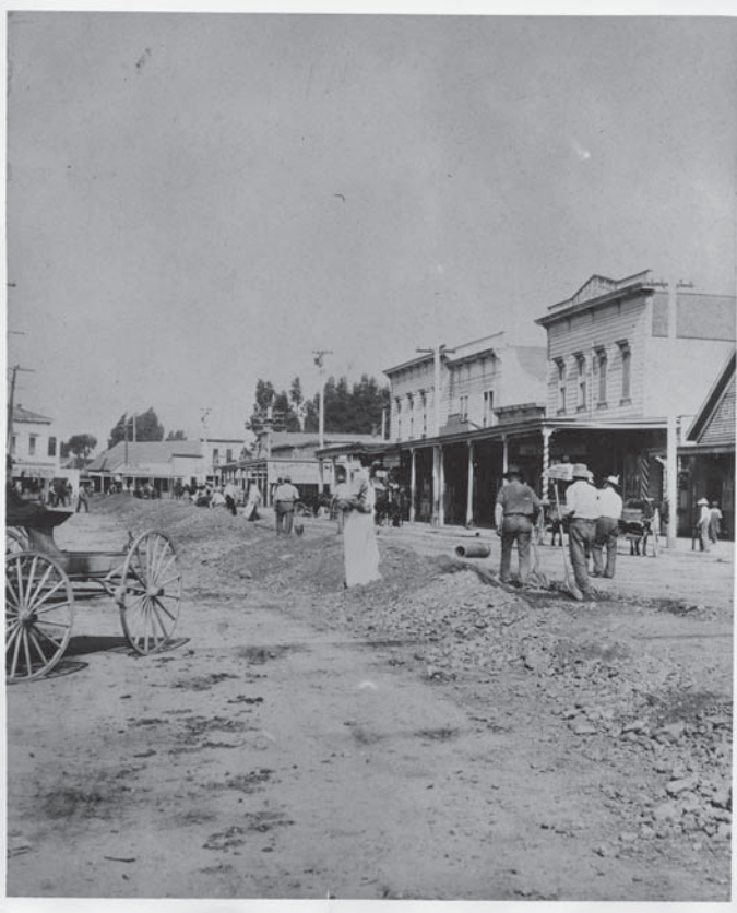
Installing sewer pipe on First Street circa 1904
