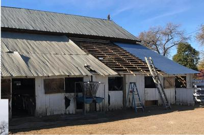
new panels blend well with the original. A light stain was brushed on the interior side of the roof panels to dull the new shine, and where new wood needed to replace old, they darkened the wood to reduce the jarring appearance of the white wood. In our first rain of the season a few of the new nail spots leaked and they came right out to patch things up. The roof is now good for many decades and maybe another century.
