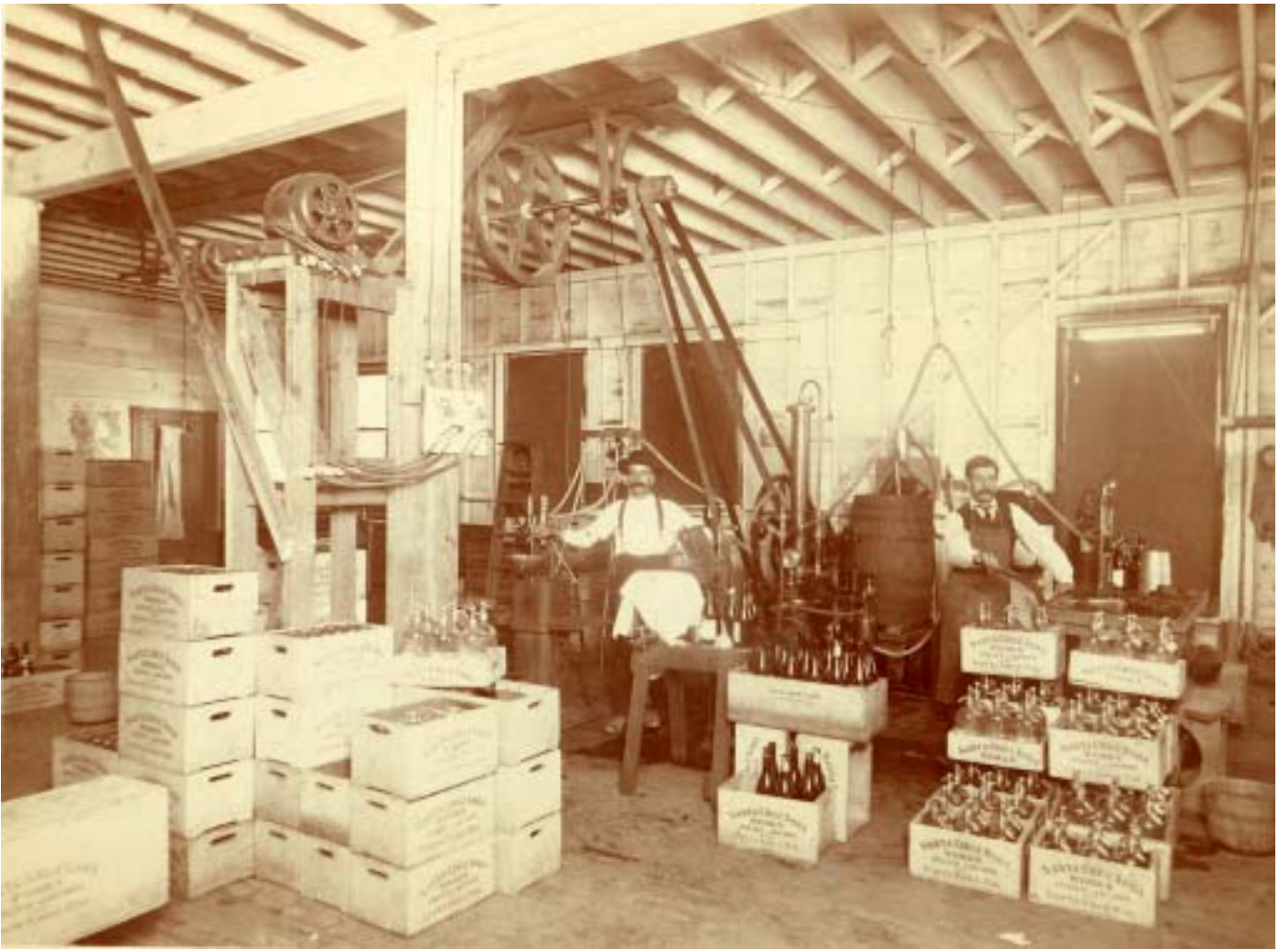
Interior of the Santa Cruz Soda Works
